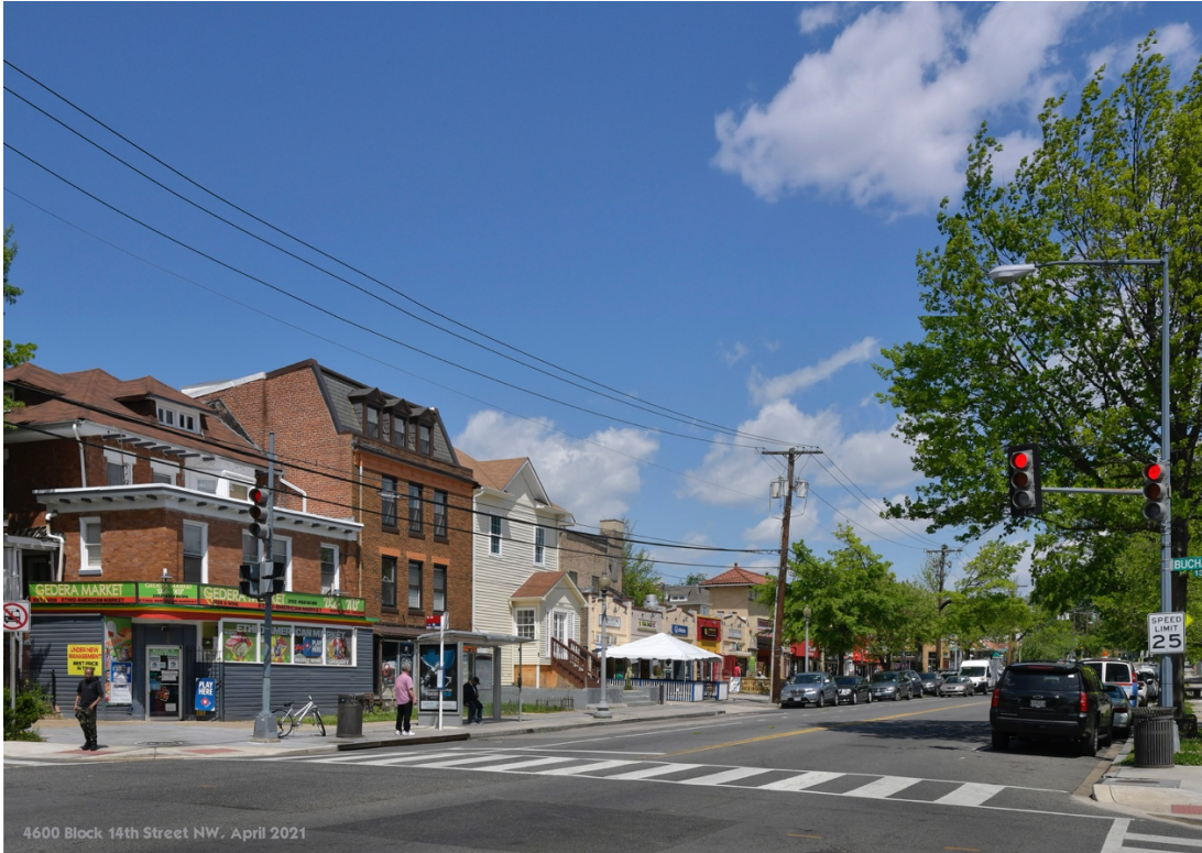
The 4600 block of 14 th Street as it currently exists (April 2021)
